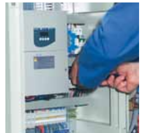
CONTROL PANEL WITH FREQUENCY IN INVERTER
